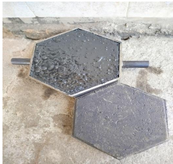
Gambar 7. Proses Pengeringan Paving.
